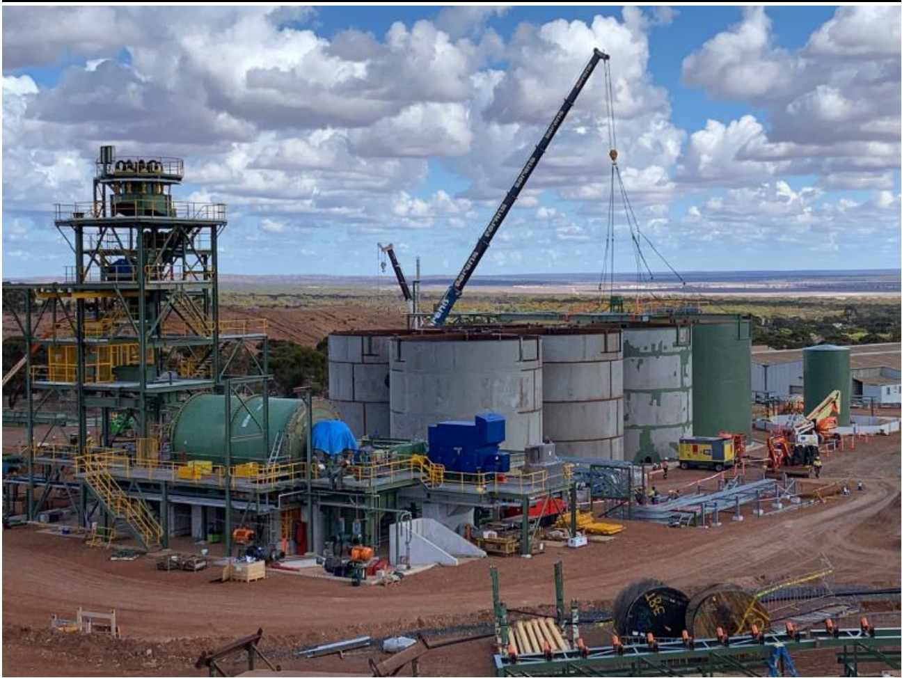
Figure 1: Construction of the processing plant at Norseman
