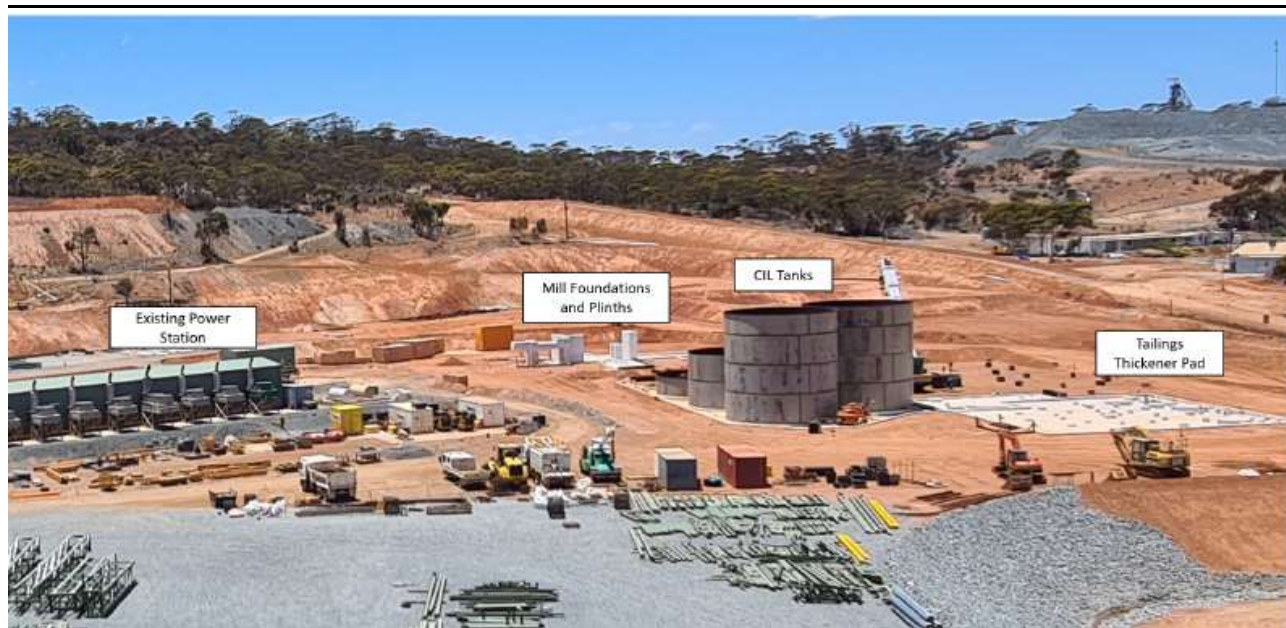
Figure 1: Construction of the processing plant at Norseman
