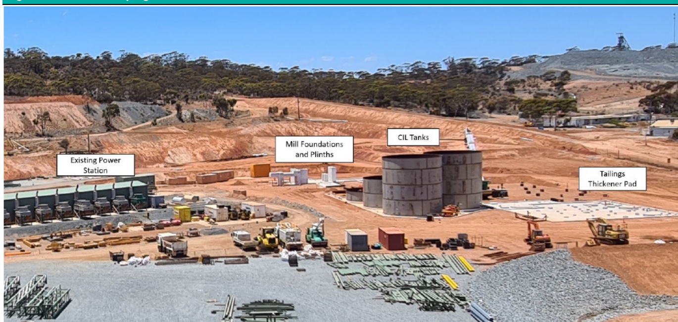
Figure 1 - Construction progress at Norseman
